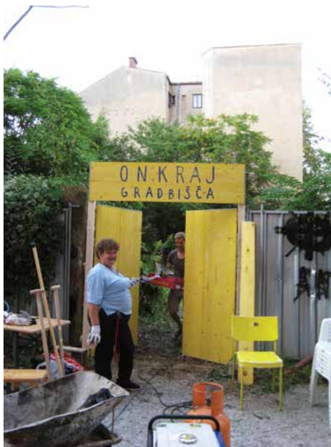
Removing part of the protective construction fence and replacing it with a door Photo by: Kud Obrat archive, August 2010
